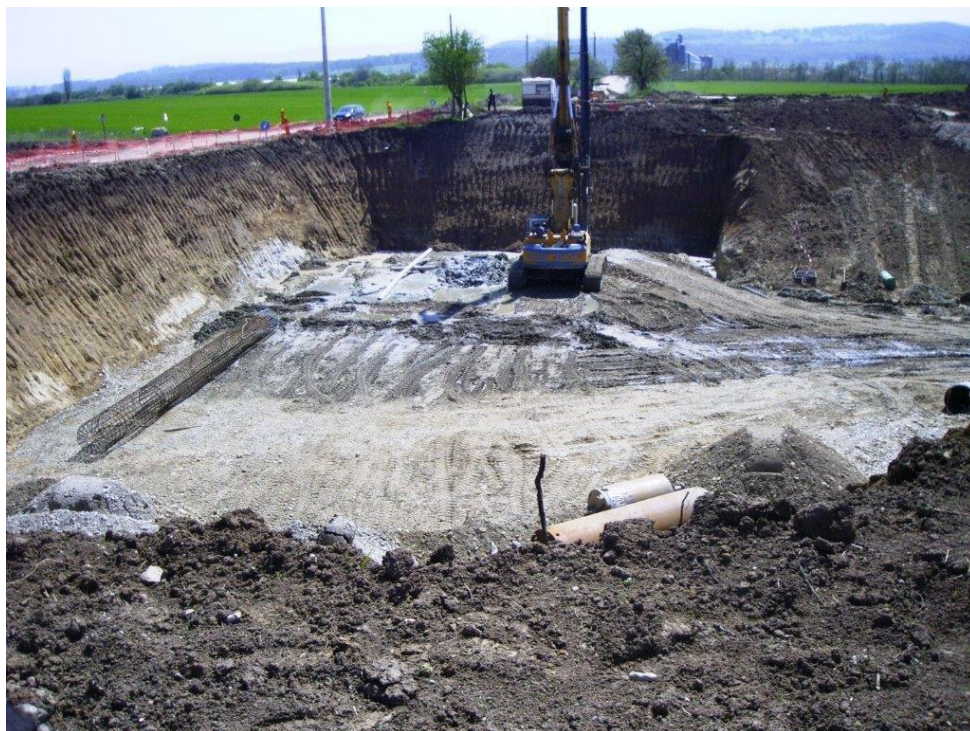
2012. Tordos - motorway construction (Photo: Klára Friedrich)
